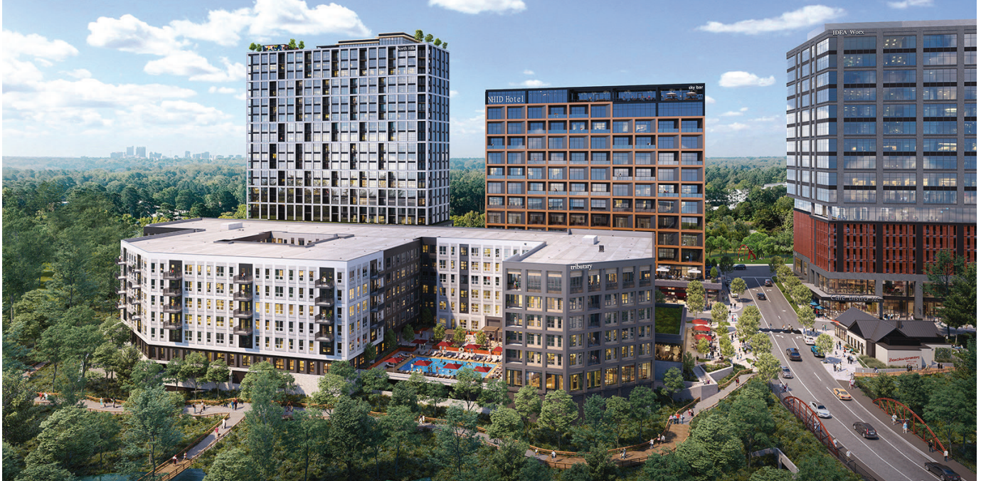
Kane Realty Corporation broke ground earlier this year on Tributary, the newest residential community within the North Hills Innovation District in Raleigh, North Carolina. Tributary will deliver 332 apartments and 6,000 square feet of ground-level retail and include a digital content creation studio.
