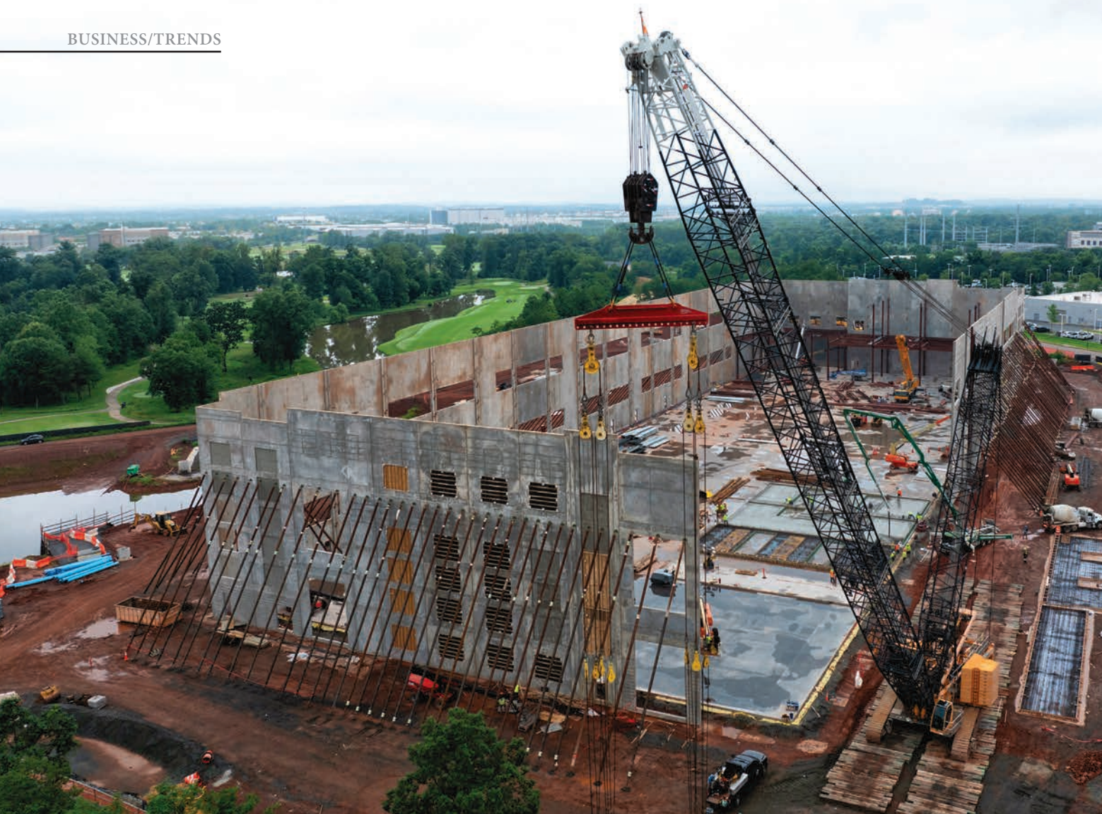
Overhead view of a data center under construction.
