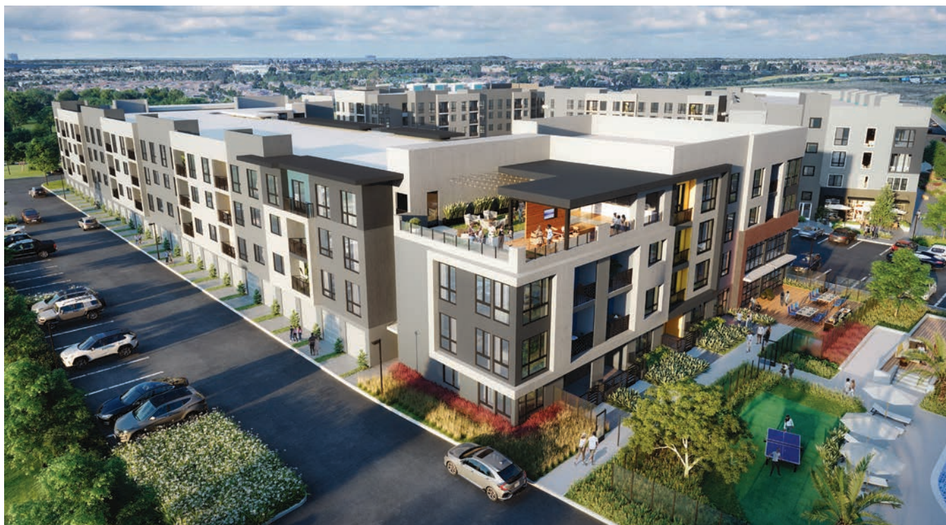
VAYA on Axia, which uses a solar array to power 278 residential units in Chula Vista, California, is representative of Ryan's commitment to sustainable development.
