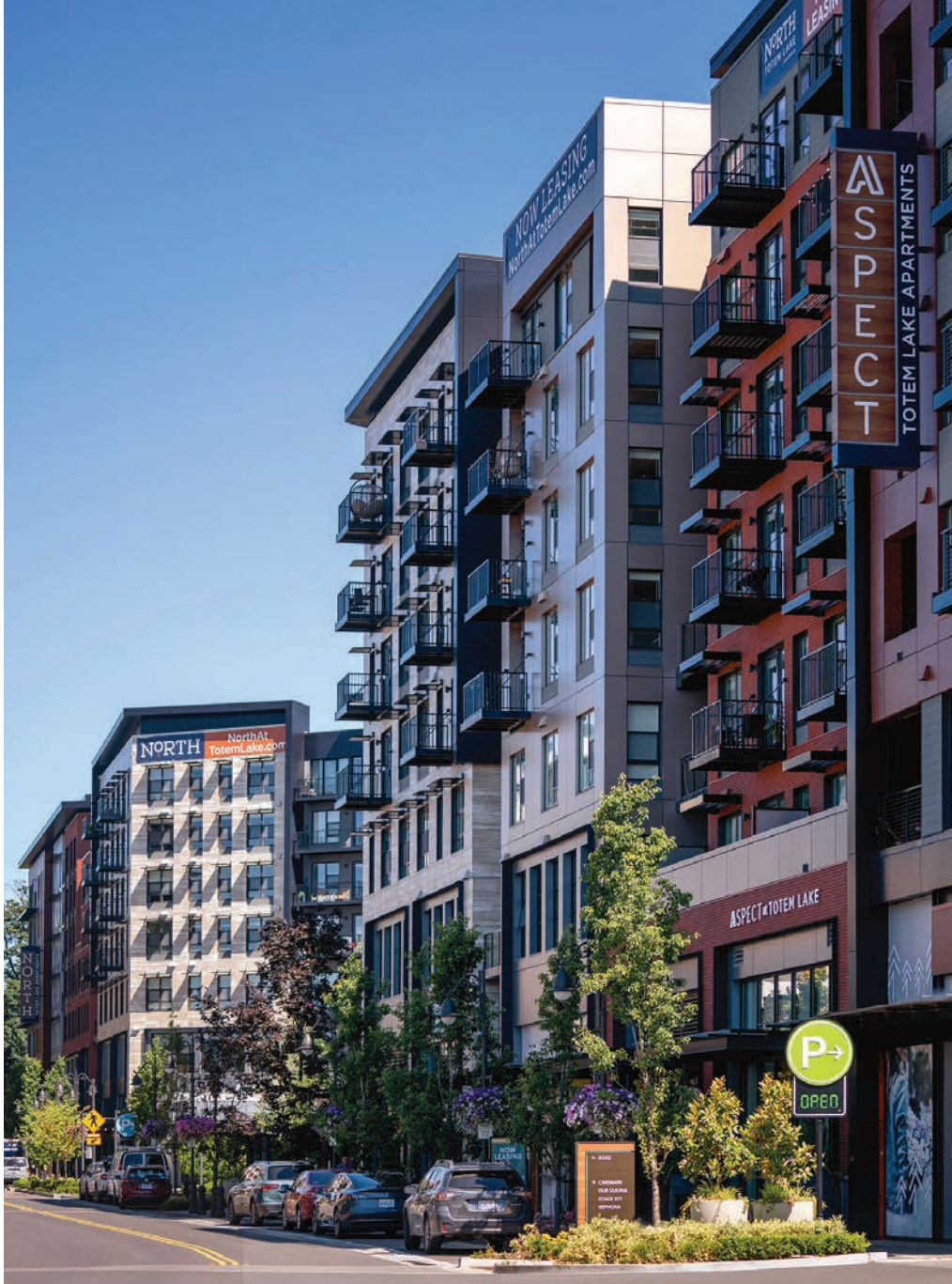
Carrier Johnson + Culture served as architect for both North and Aspect, two of the three residential communities within the Village at Totem Lake.
