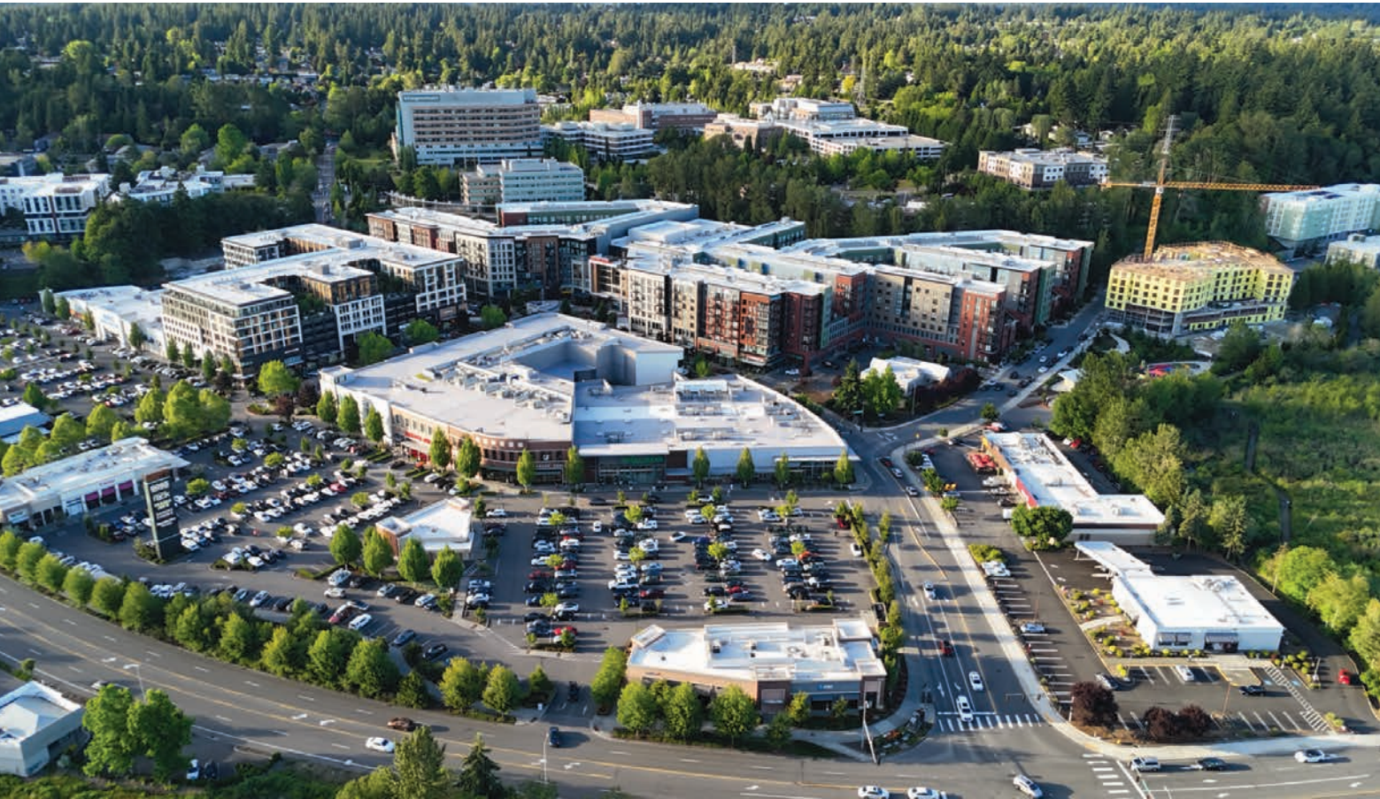
An aerial view of The Village at Totem Lake, a 21-acre, $670 million transformation of a former enclosed mall into a mixed-use urban village outside of Seattle.
