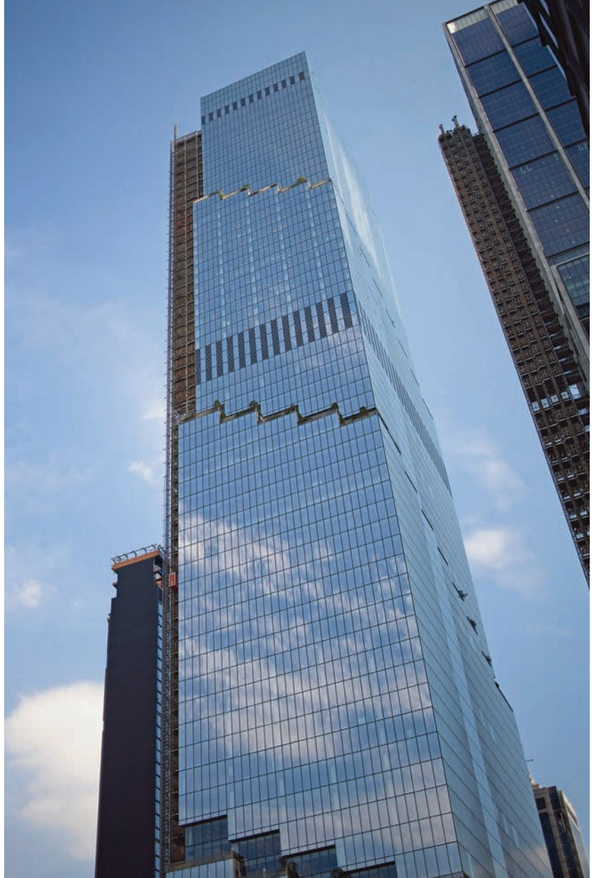
Building operations at The Spiral are coordinated through an integrated platform that connects environmental controls, energy management and irrigation systems.
