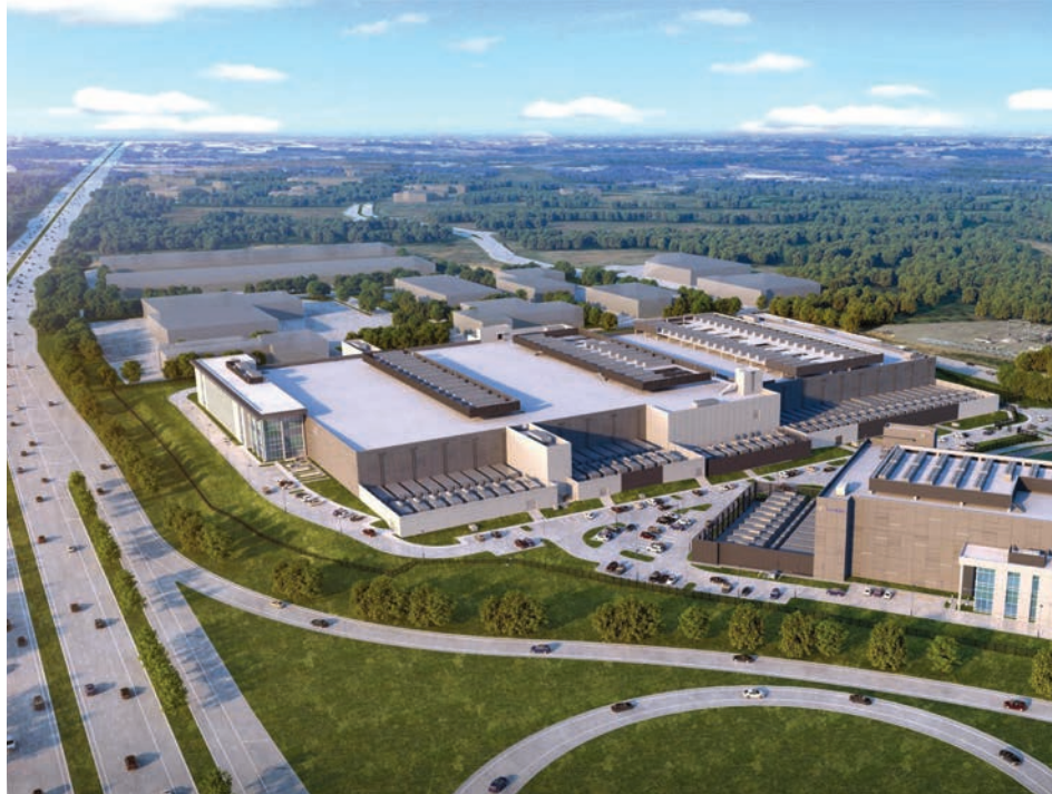
It is critical to account for evolving power needs, especially with large, master-planned data center campuses and AI campuses.
