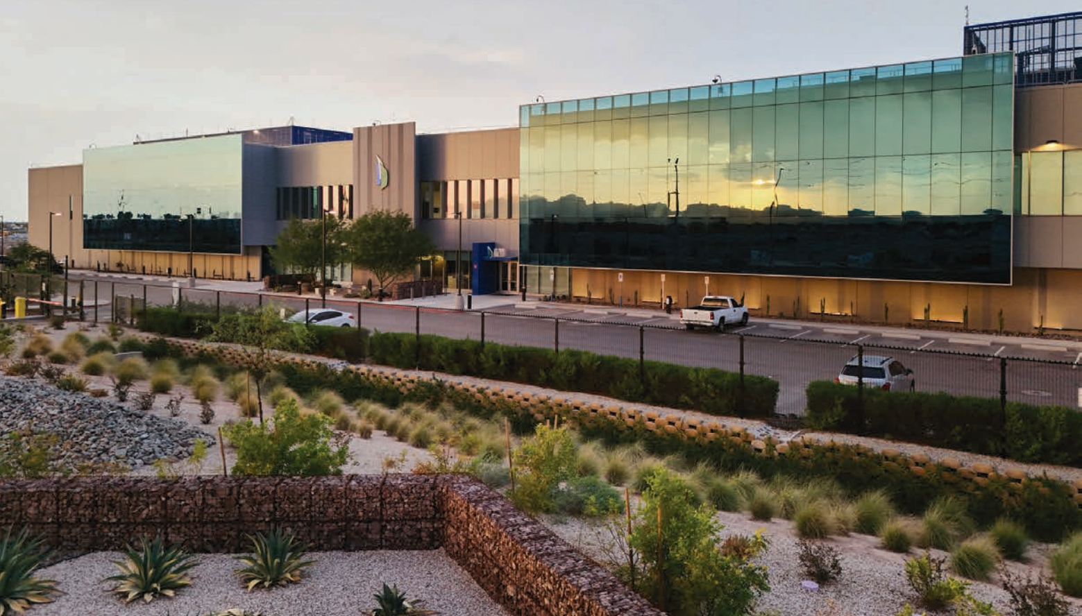
The Vantage Data Centers AZ1 campus in Goodyear, Arizona, will have a combined capacity of 176 megawatts.
